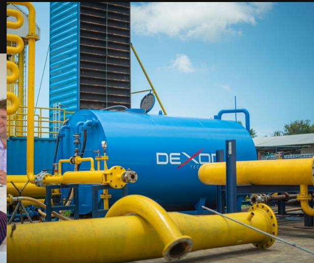
Construction Fabrication and Maintenance
